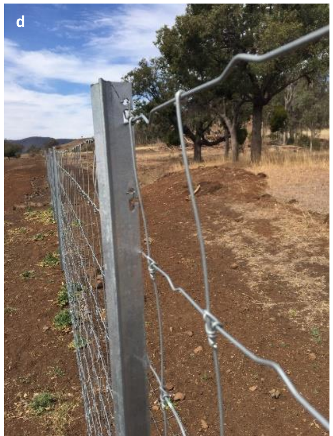
Figure 14. A Liverpool Plains, NSW, fence. Note the absence of plain wires (top, bottom and belly), rather, the mesh netting is tied directly to the posts and the apron is hinged.
