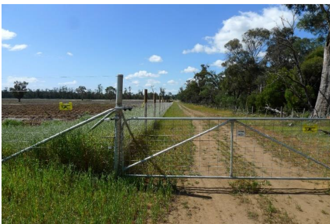
Figure 15. The Cressy, Tasmania, fallow deer exclusion fence. Note the chicken-wire netting up to 1.5 m and the two widely spaced horizontal wires at the top of the fence. This netting enabled deer to push through the fence and the wide spacing of the wires allowed them to jump the fence.
