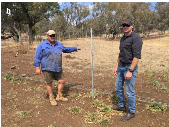
Figure 14. A Liverpool Plains, NSW, fence. Note the absence of plain wires (top, bottom and belly), rather, the mesh netting is tied directly to the posts and the apron is hinged.
