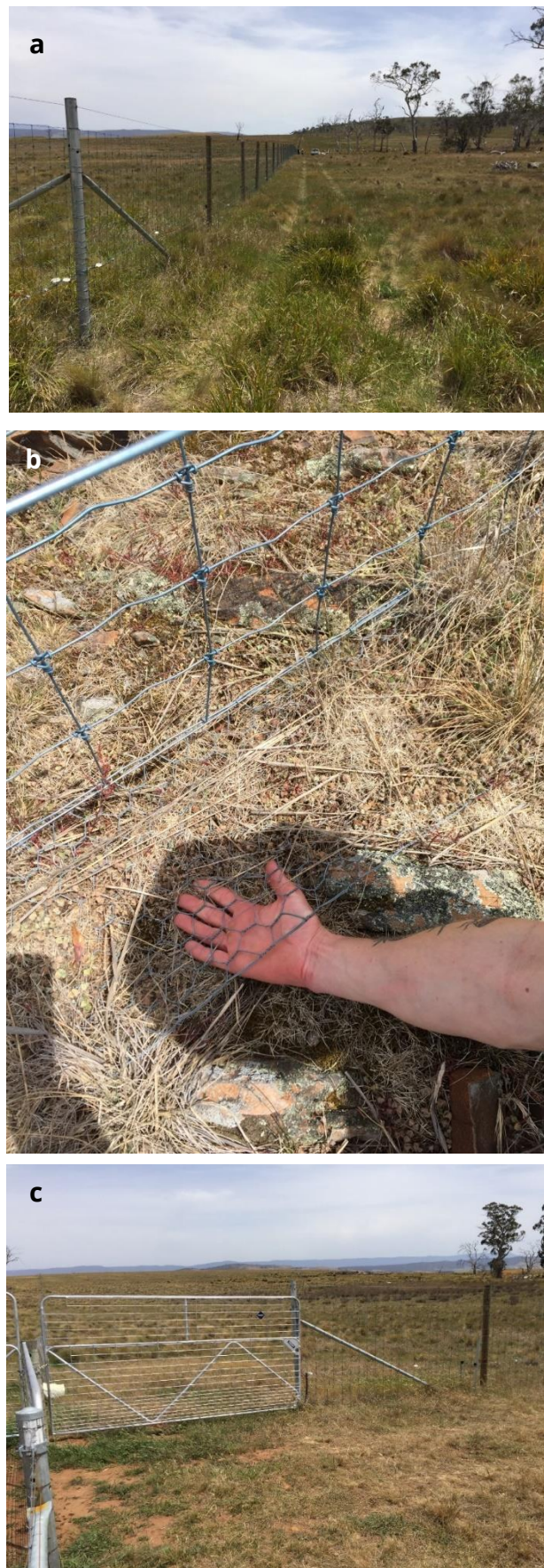
Figure 13. The Midlands, Tasmania, fence. Note the electric outriggers ('hotwires') inside and outside the fence 50 cm above ground level and (b) the 30 cm apron extending out from the fence.
