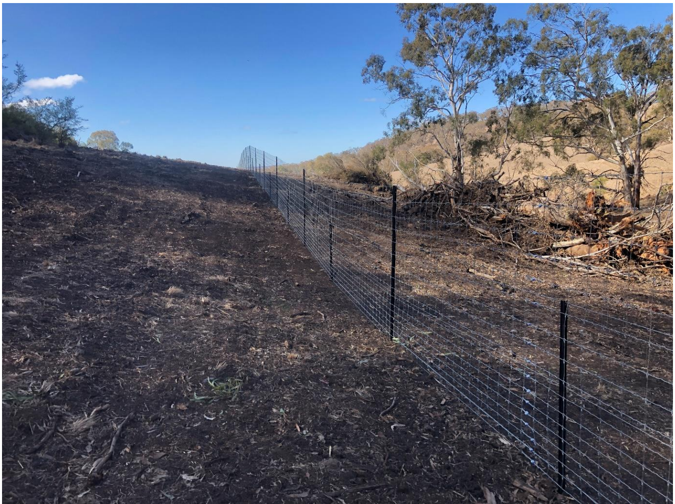
Figure 5. Prior to erecting this deer exclusion fence, the fence line was cleared (i.e. trees pushed aside) and levelled by a bulldozer.
