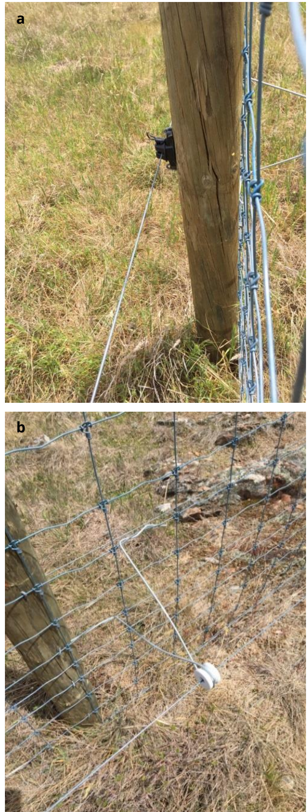
Figure 7. Examples of electric outriggers on (a) the inside and (b) the outside of a deer exclusion fence. Both outriggers are 50 cm above the ground, and the outside wire is 30 cm out from the fence. The objective of the inside outrigger is to prevent livestock (in this case sheep and cattle) from pressing against the fence. The outside outrigger prevents deer, macropods and livestock from pushing against the fence.
