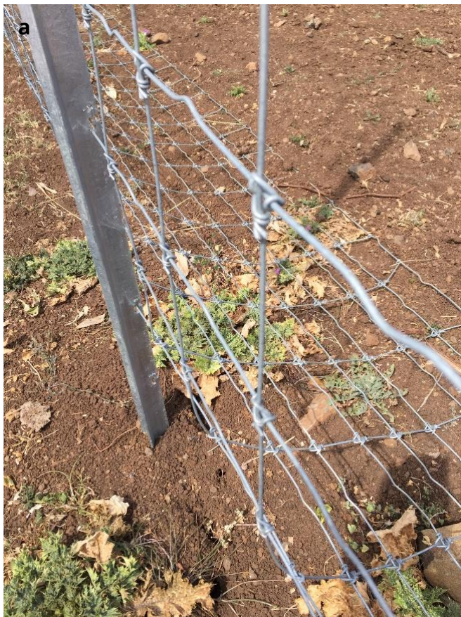
Figure 6. Two examples of 30 cm aprons on deer exclusion fences. In (a), the bottom of the netting flares out. In (b), the chicken wire netting has been tied to the plain bottom wire at the base of the deer netting.
