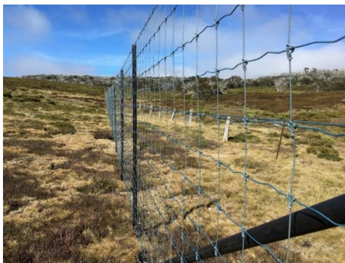
Figure 16. The Maisie's Plot sambar deer and horse exclusion fence in the Bogong High Plains, Victoria. The upper right figure shows a gate allowing people to access the plot, and horses that become trapped in the plot to exit it. Source: Elaine Thomas, Parks Victoria.
