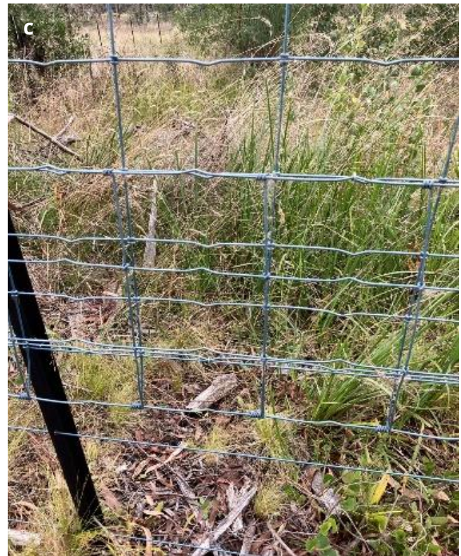
Figure 18. The partial sambar and fallow deer exclusion fence at Pheasant Creek Flora Reserve, North East Victoria: (a) a corner of the fence, (b) three-pin anchor (at gate post), (c) star post with raised apron, (d) double gate that can be opened to allow animals inside the fence to be mustered out, and (e) tree-fall over the fence requiring the tree to be cut up and the fence repaired
